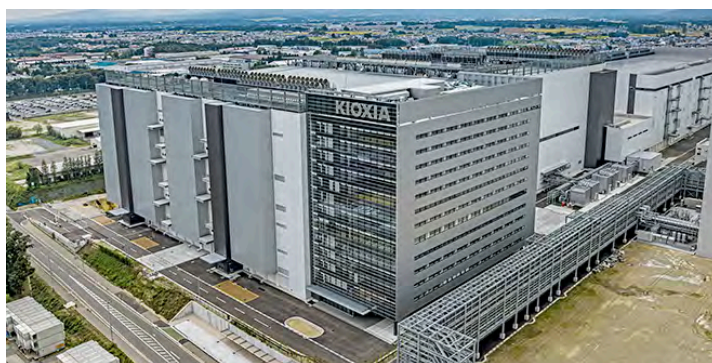
Fab2 and management building at Kioxia Iwate Corporation
